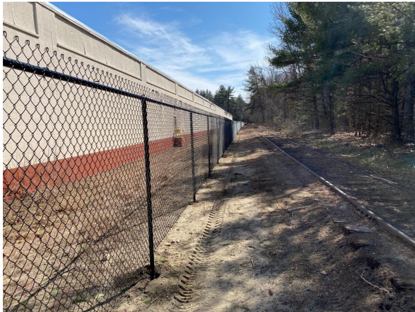
The newly installed fence behind Sterilite
