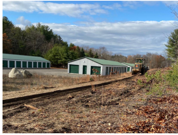
Pulling a long section of rail back to the staging area at Depot Street.
