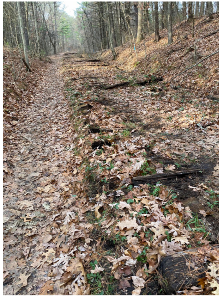
The ties remaining after the rails have been removed.
