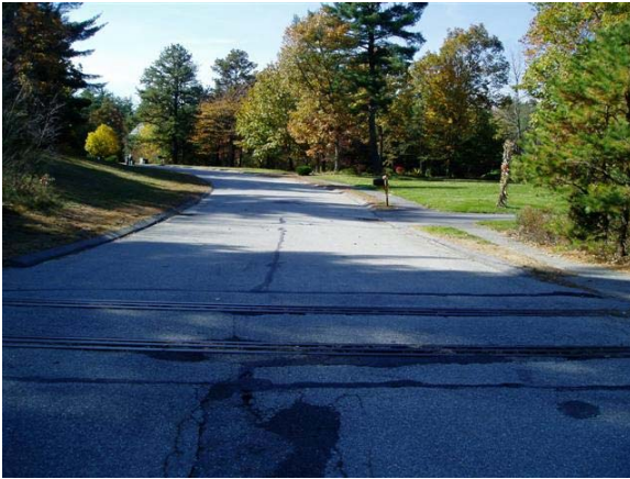
Figure 39: Crosswinds Drive Northern Crossing
