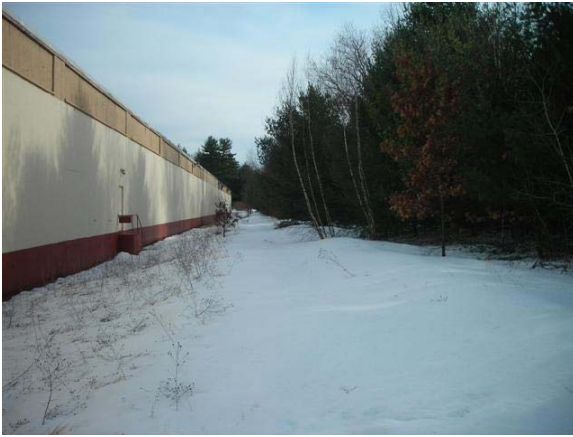
Figure 80: Rear of Sterilite Property
