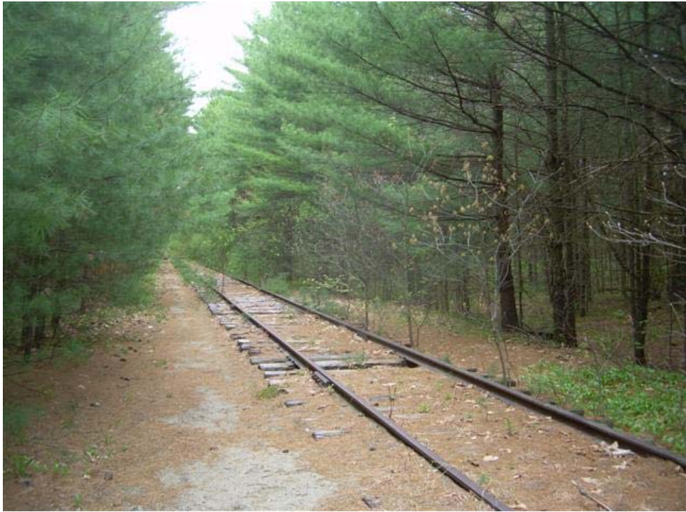
PHOTO 3: Existing Railroad Corridor Looking North
