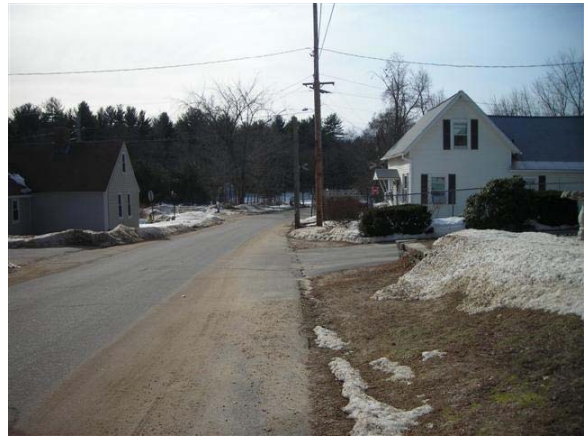
Figure 53: Depot Street Looking West
