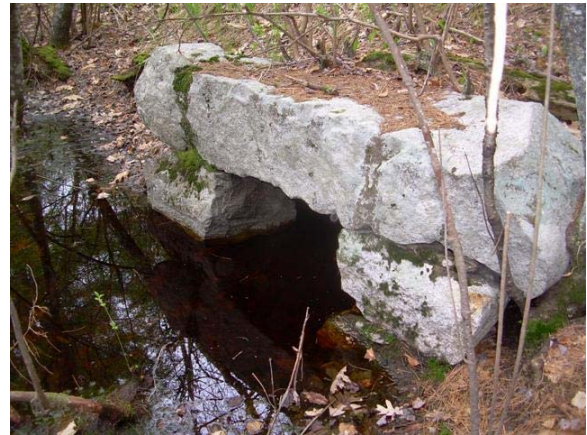
Figure 43: Culvert No. 42.09 North of Crosswinds Drive
