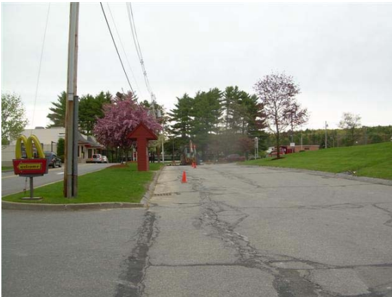
Figure 65: Access Road Between Harbor Village Shopping Center and McDonald's Looking East
