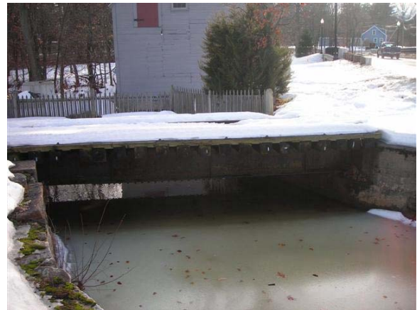
Figure 49: Bridge No. 44.13 Side View
