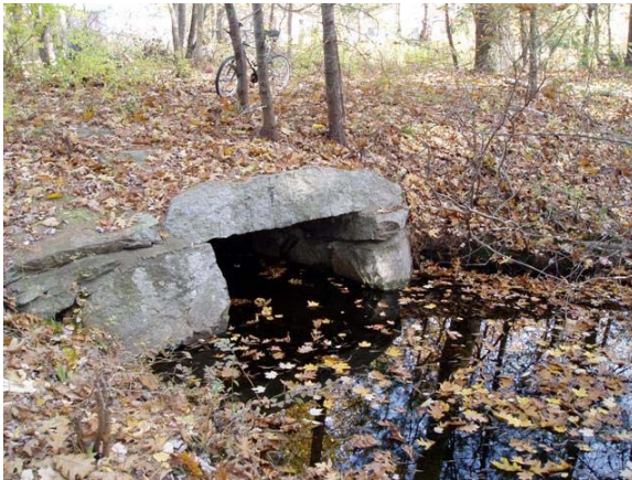
Figure 42: Culvert No. 44.35 South of Old Meetinghouse Road
