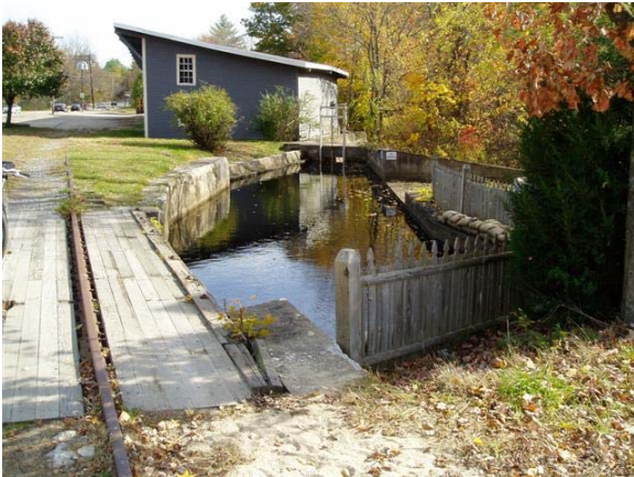
Figure 18: Peterborough and Shirley Railroad Bridge Over Grist Mill Sluiceway
