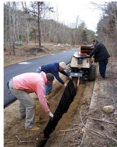
Figure 20: Root Barrier Installation
