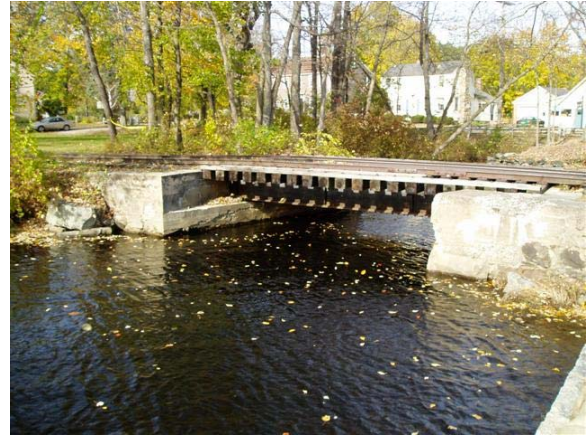
Figure 47: Bridge No. 44.17 Side View
