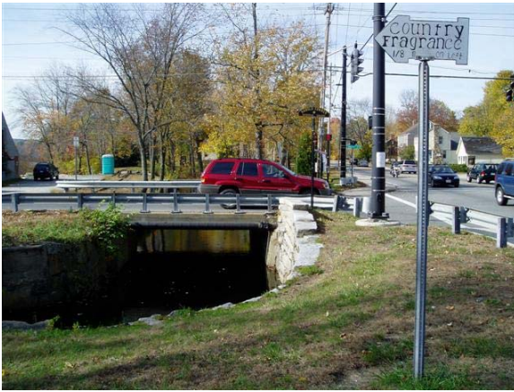
Figure 57: Route 119 Looking North South of South Road
