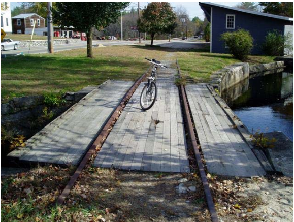
Figure 48: Bridge No. 44.13 Looking South
