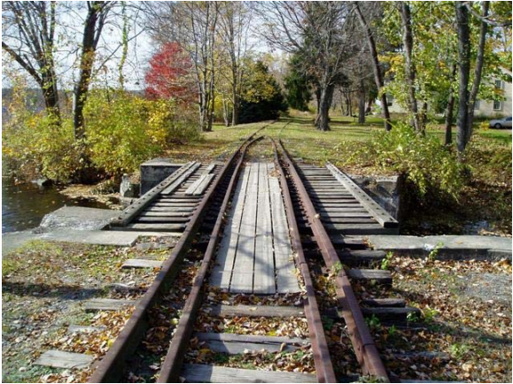
Figure 46: Bridge No. 44.17 Looking North
