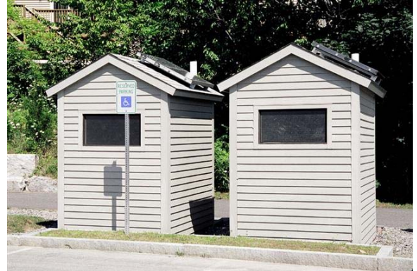
Figure 88: Example Comfort Facilities Nashua River Rail Trail
