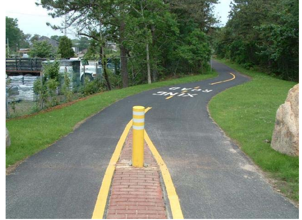
Figure 31: Narrow Median Application
