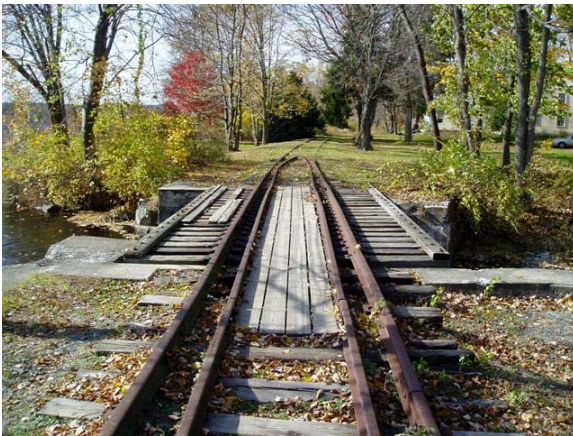
Figure 55: Railroad Corridor Behind Reed Homestead
